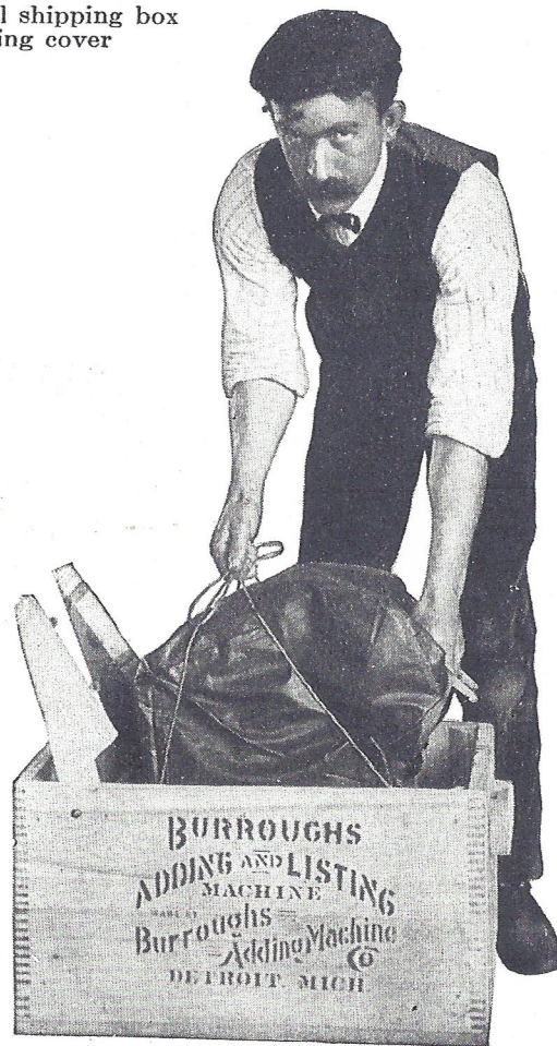
Fig. 3 Lift the machine carefully out of the box by means of the cords
